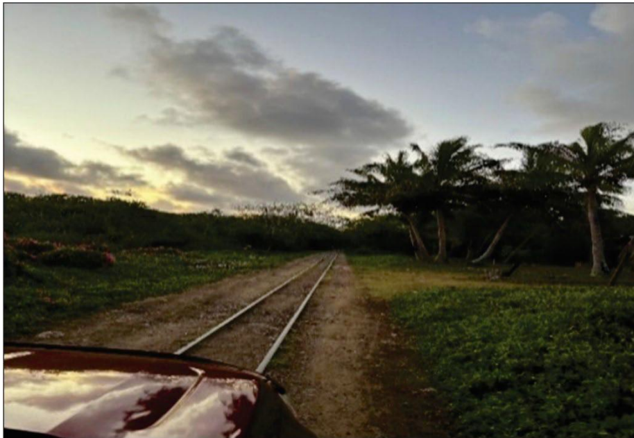
Figure 4. Tramline at Muanivatu is often used instead of the road which is often in a poor state of repair.
