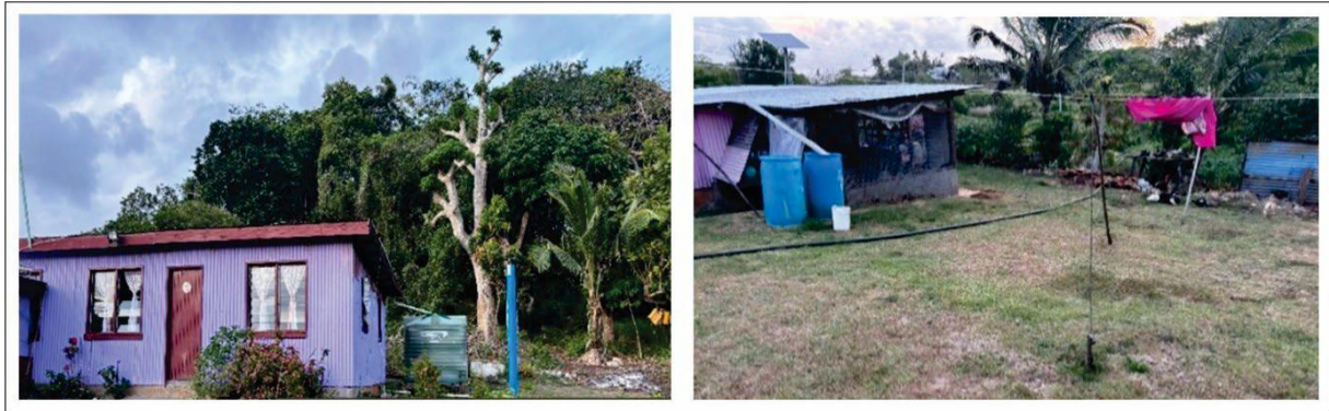
Figure 5. Muanivatu water storage – rainwater tanks linked to roof catchment (left) and moveable storage drums linked opportunistically to roofs (right).
