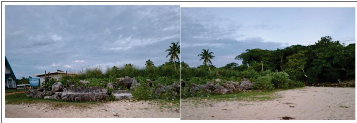
Figure 14. Seawall constructed at Malomalo by the Fiji Government.
