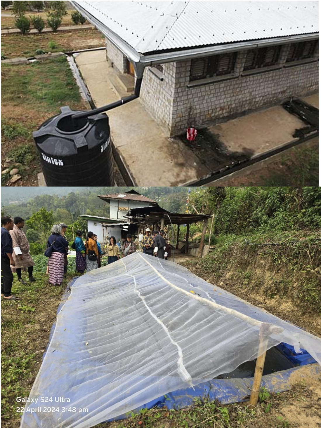
Figure 21: Rain water harvesting, using a plastic-lined pond to store water
