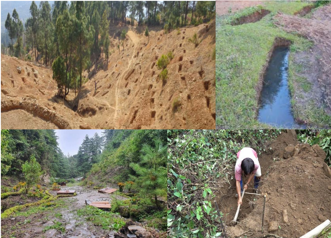
Figure 23: Spring shed recharge trenches (Source: Down to Earth and nature based solutions, Bhutan)
