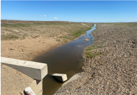
Water channel to divert water flow
