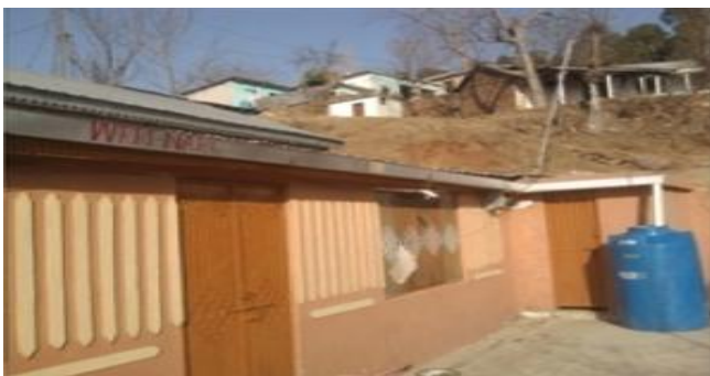
Figure 3: Roof top rainwater harvesting
