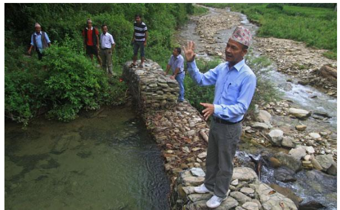
Figure 1: Loose Rocks Check Dam.
