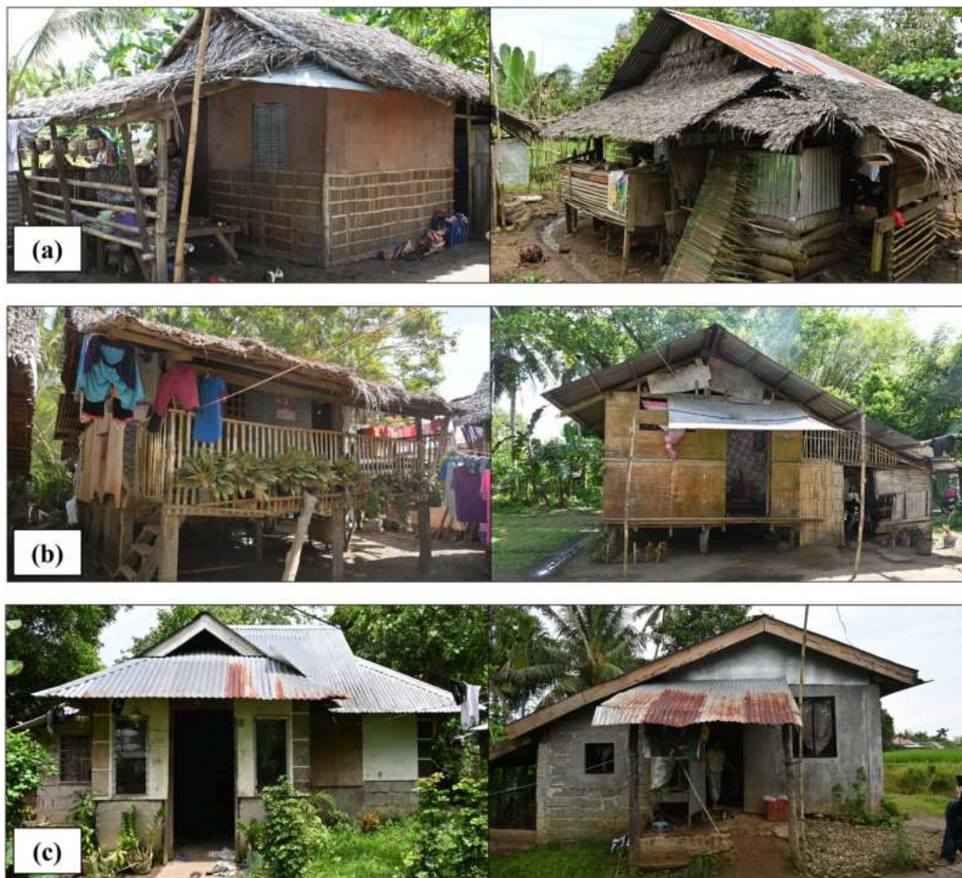
Fig. 3. Building typologies identified for localised vulnerability functions. (a) Light material, (b) elevated light material, and (c) concrete structures.
