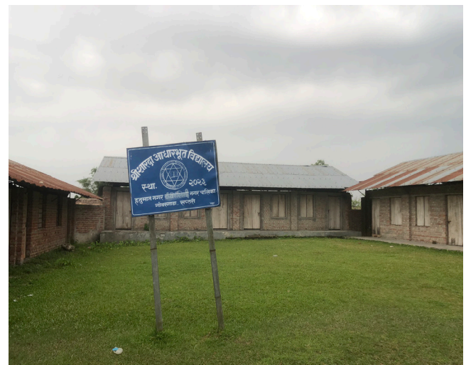
Figure 2. A primary school in Gobargada village adjacent to Koshi River
