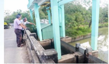
Surveying infrastructure in flood-prone areas.
