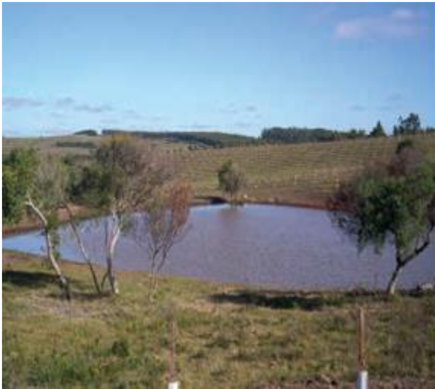
Figure 10: Pond for Groundwater recharge
