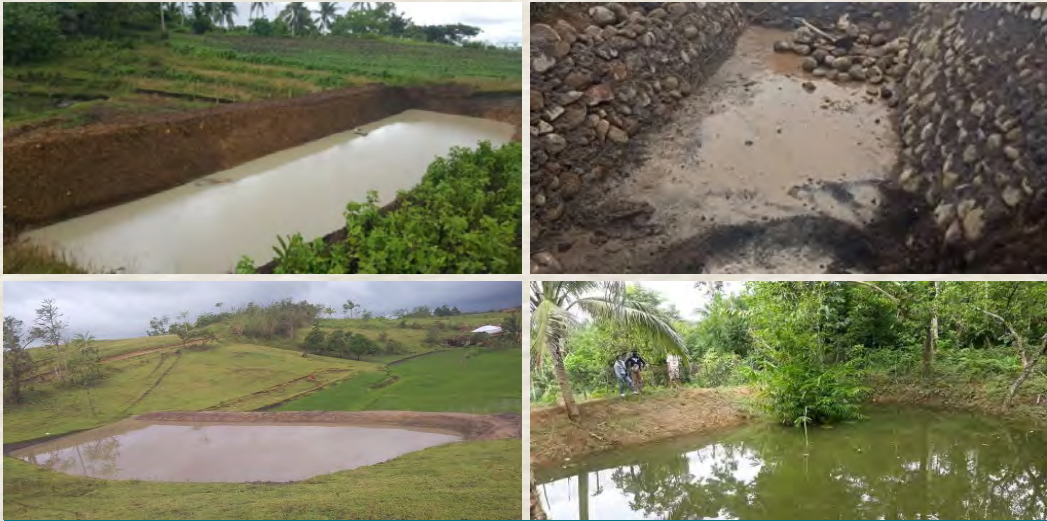
Figure 17. Rainwater harvesting ponds differ in each site in terms of size and structure. These were established by the upland farmers, harnessing their collection action (bayanihan) (Photo credit: CBA2019-01NSY Landicho)
