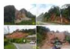
(a) a shallow translation of rockslide (b) a shallow translation of debris slide at the road side, (c) and (d) deep-seated rotational slides. As an aside, the movement direction.
