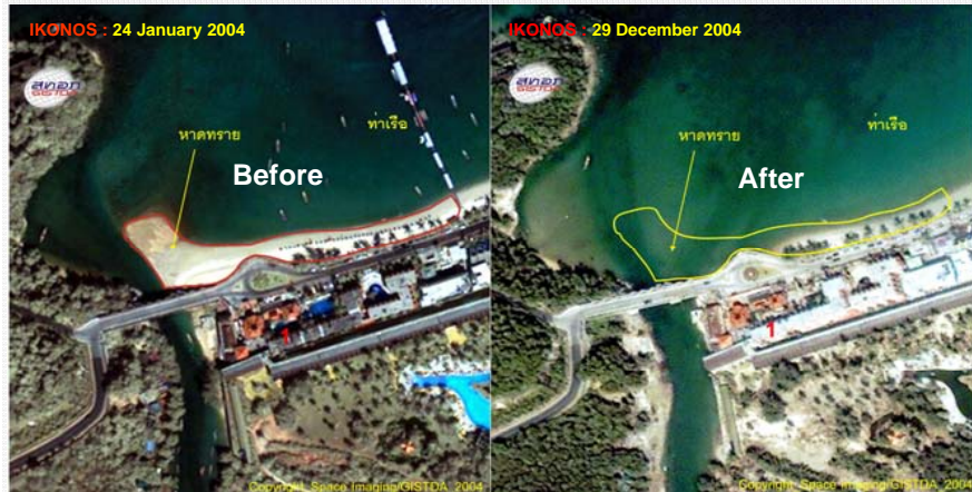
Destroyed Areas, Buildings, Roads, Beaches, Port and Flooded areas Patong Beach, Phuket
