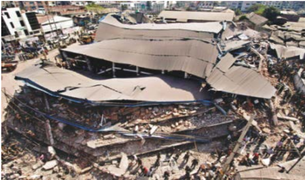
Figure 16. Phoenix garments factory building collapse 2006. Image: Anisur Rahman, courtesy of The Daily Star
