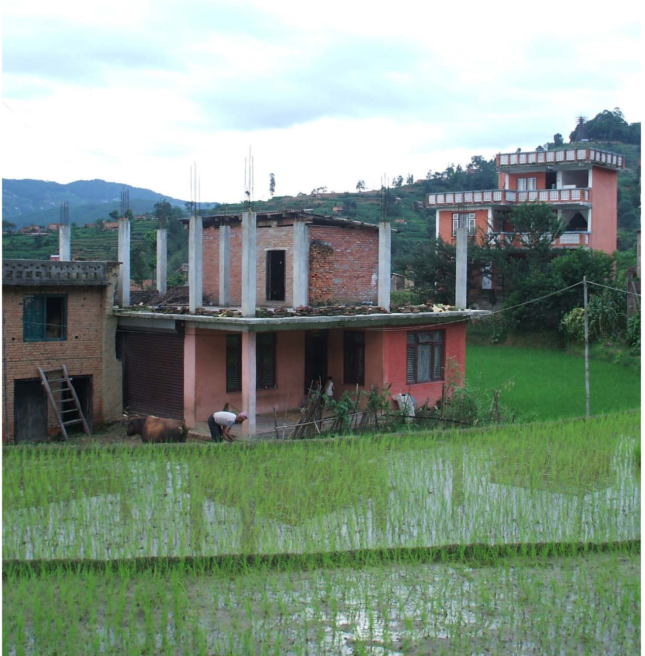
Figure 20. Housing construction, Nepal
