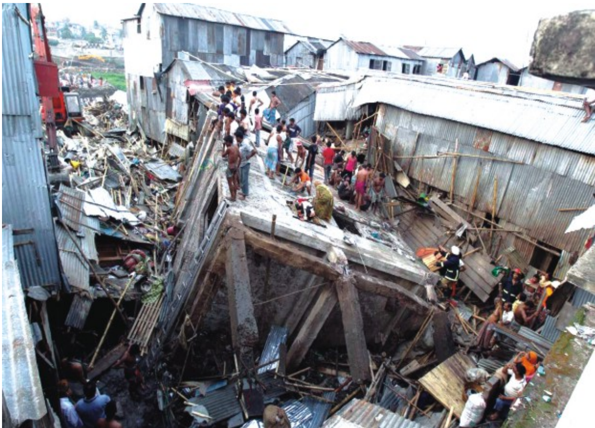
Figure 14. Begunbari building collapse 2010. Image courtesy of The Daily Star
