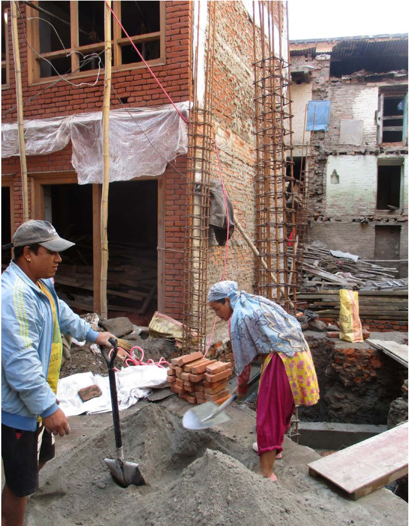
Figure 2. Construction site, Nepal
