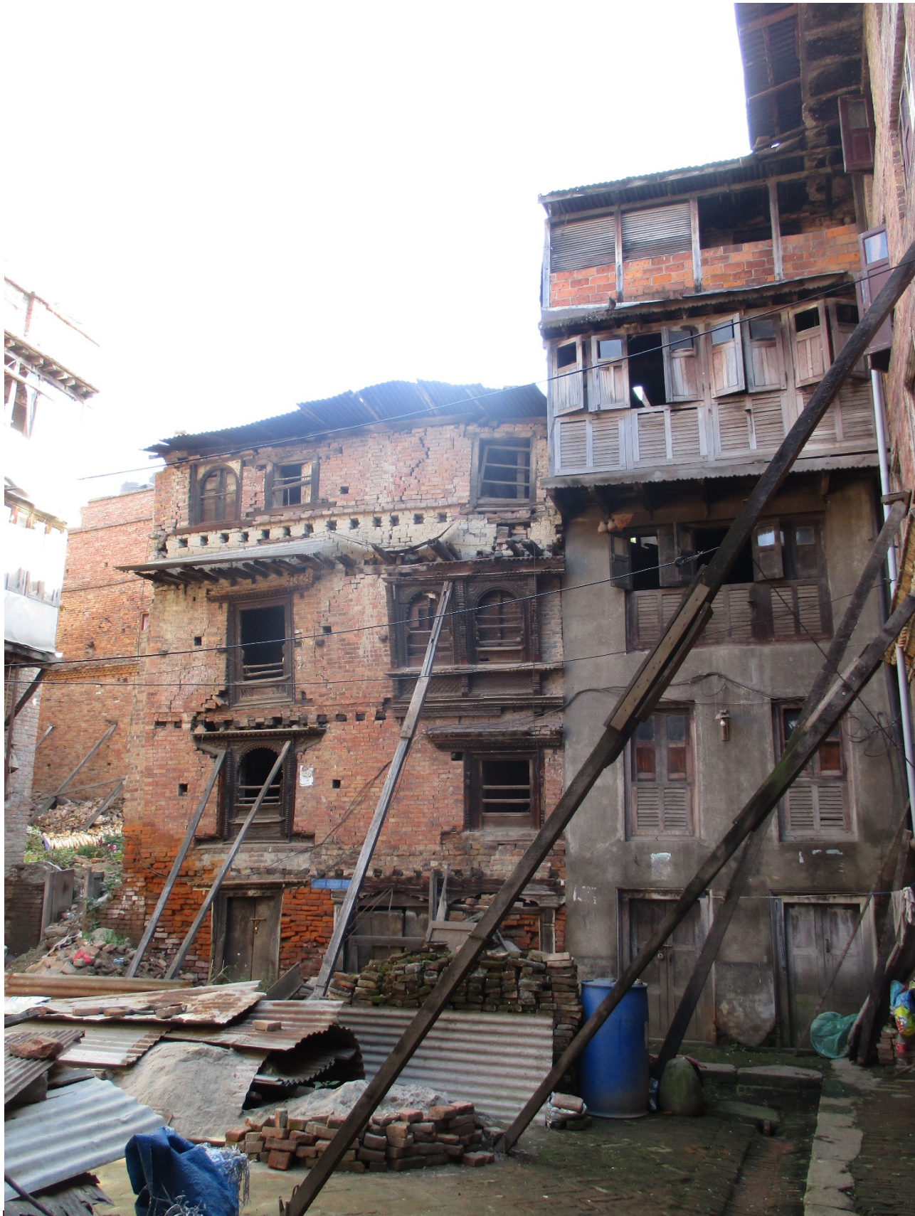
Figure 31. Old and deteriorating buildings in Kathmandu, Nepal; note how the buildings are buttressed to prevent toppling
