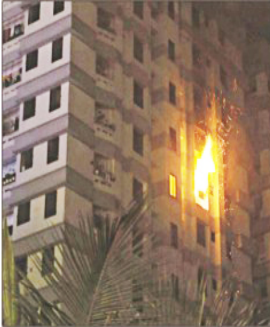
Figure 13. Building fire in Japan Garden City 2010, Image courtesy of The Daily Star
