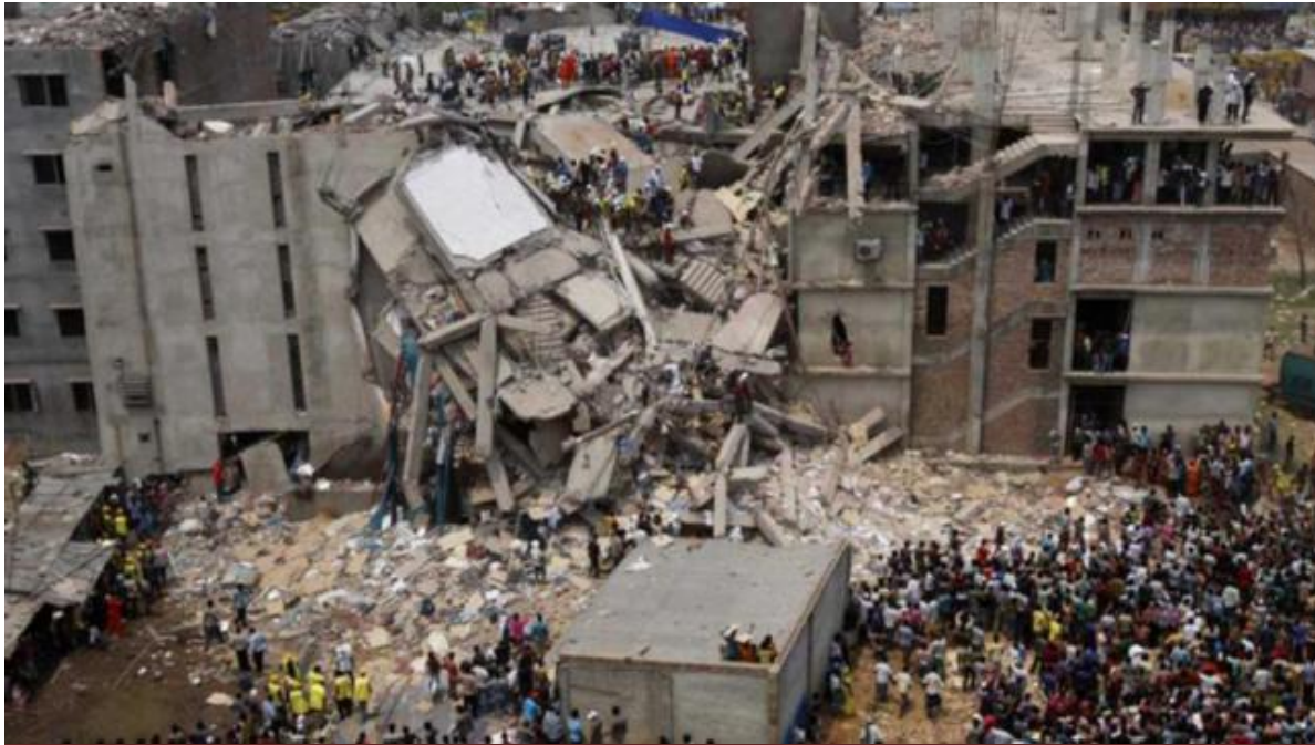
Figure 17. Rana Plaza building collapse 2013. Image courtesy of The Daily Star
