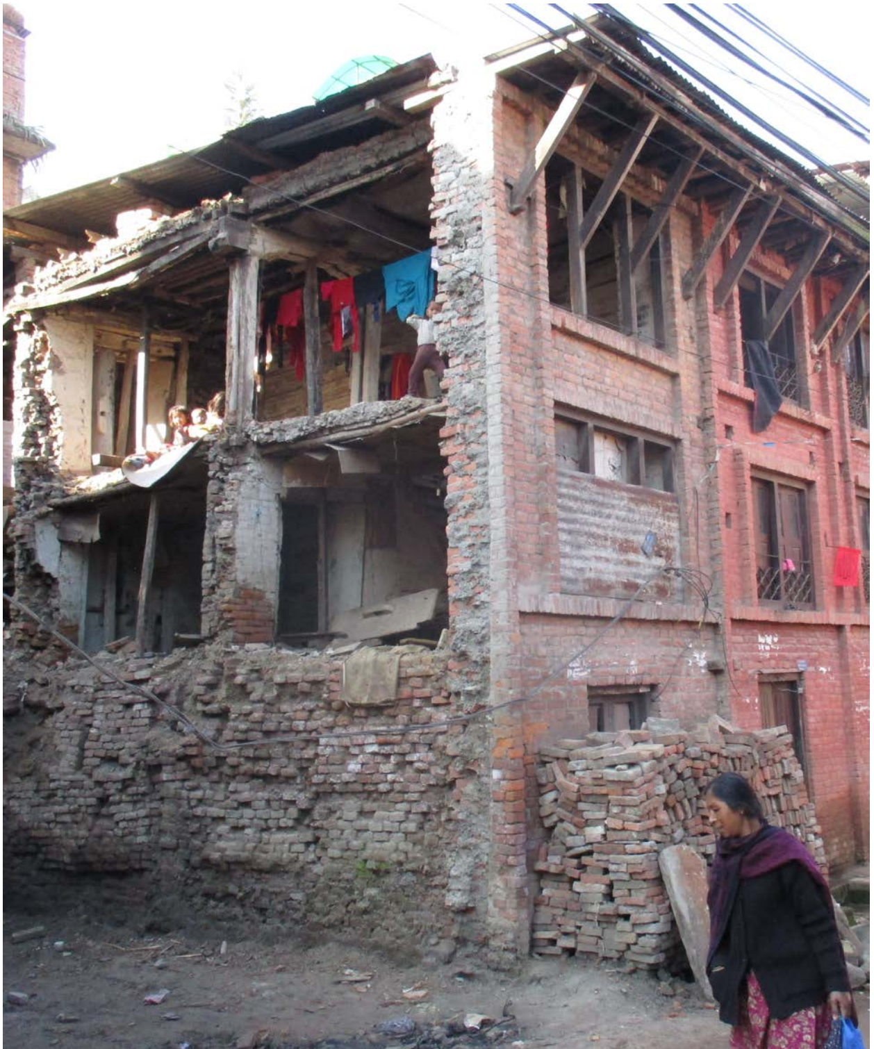
Figure 29. A building damaged by the 2015 Gorkha earthquakes in Nepal
