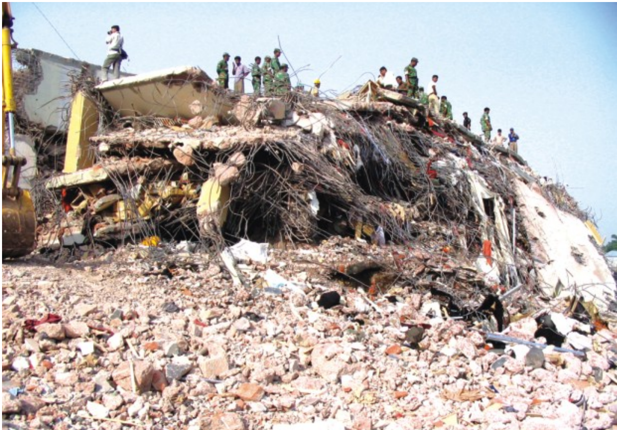
Figure 15. Spectrum sweater factory building collapse 2005. Image: Zahedul I Khan, courtesy of The Daily Star
