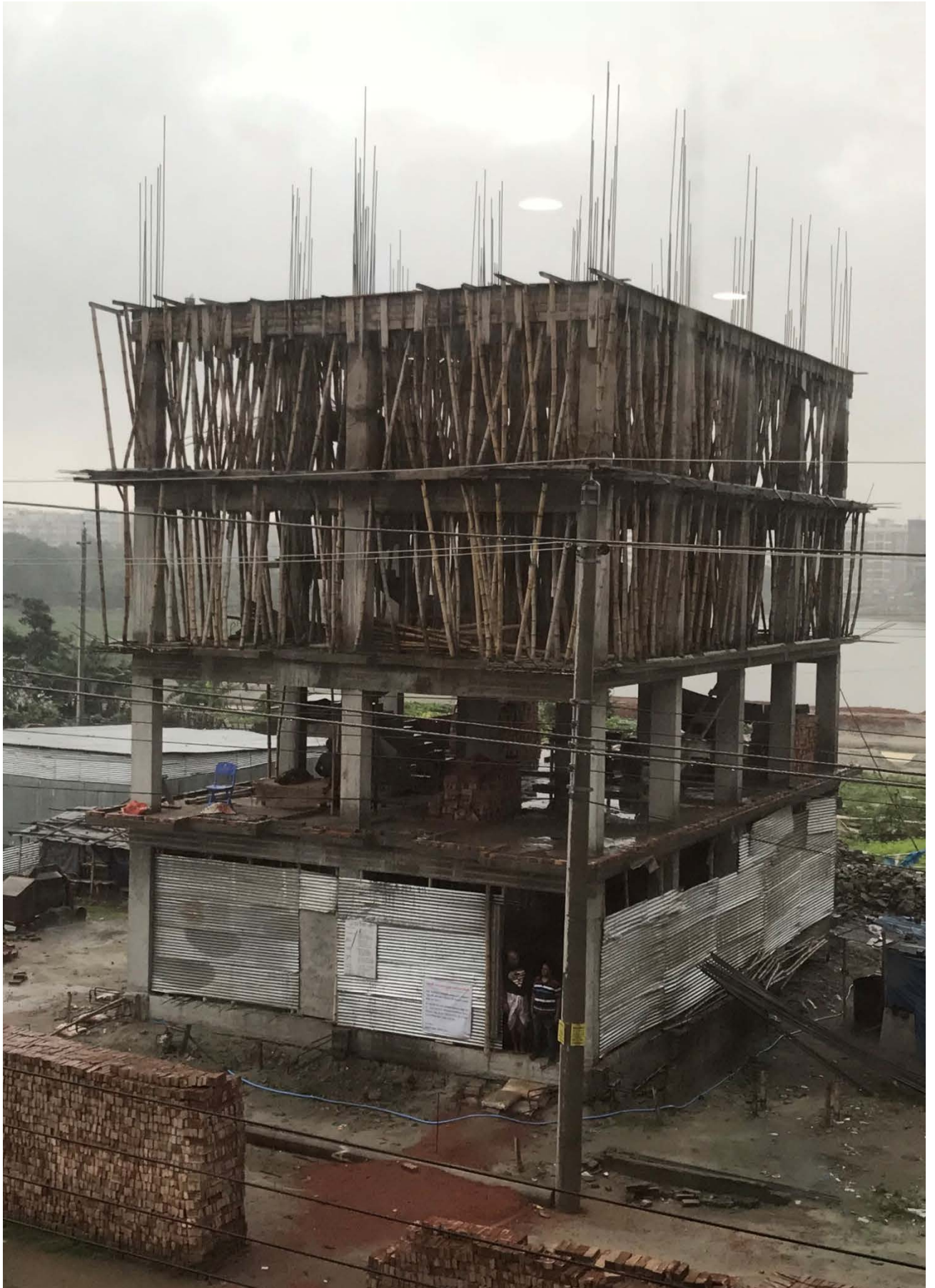
Figure 1. Construction Site, Bangladesh
