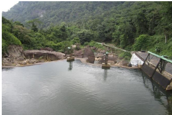
Plate 9.6: Plate Diversion and pond behind the weir
