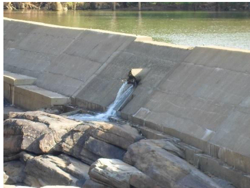
Plate 9.3: Unsatisfactory environmental flow
