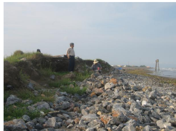
Fig. 6. Former seadike in Hai Hau
