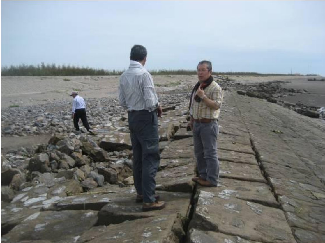
Fig 5. The investigation the problem of sea dike erosion in Hai Hau, Nam Dinh province
