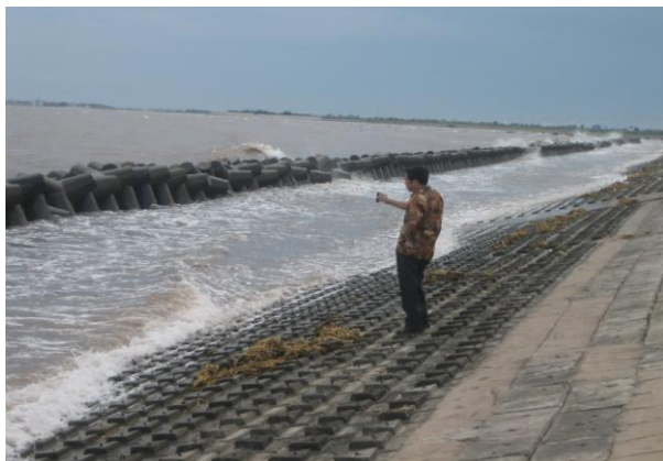
Fig. 11. New concrete dike
