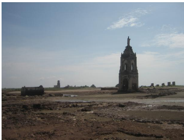
Fig. 5. Land loss due to erosion in Hai Ly
