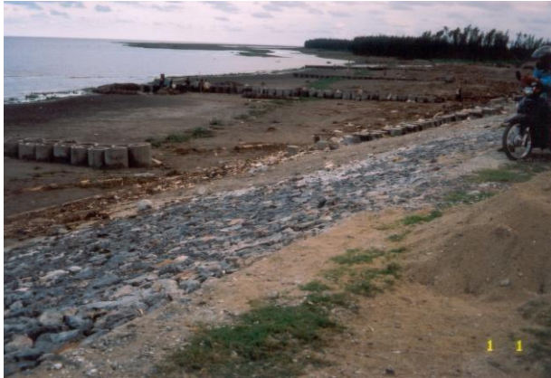
Fig. 9. Revetment and groins
