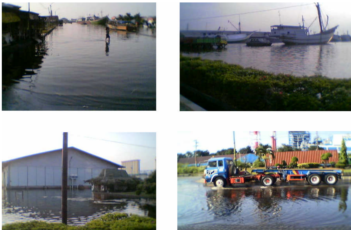
Figure 6. Inundation in the Port of Tanjung Mas
