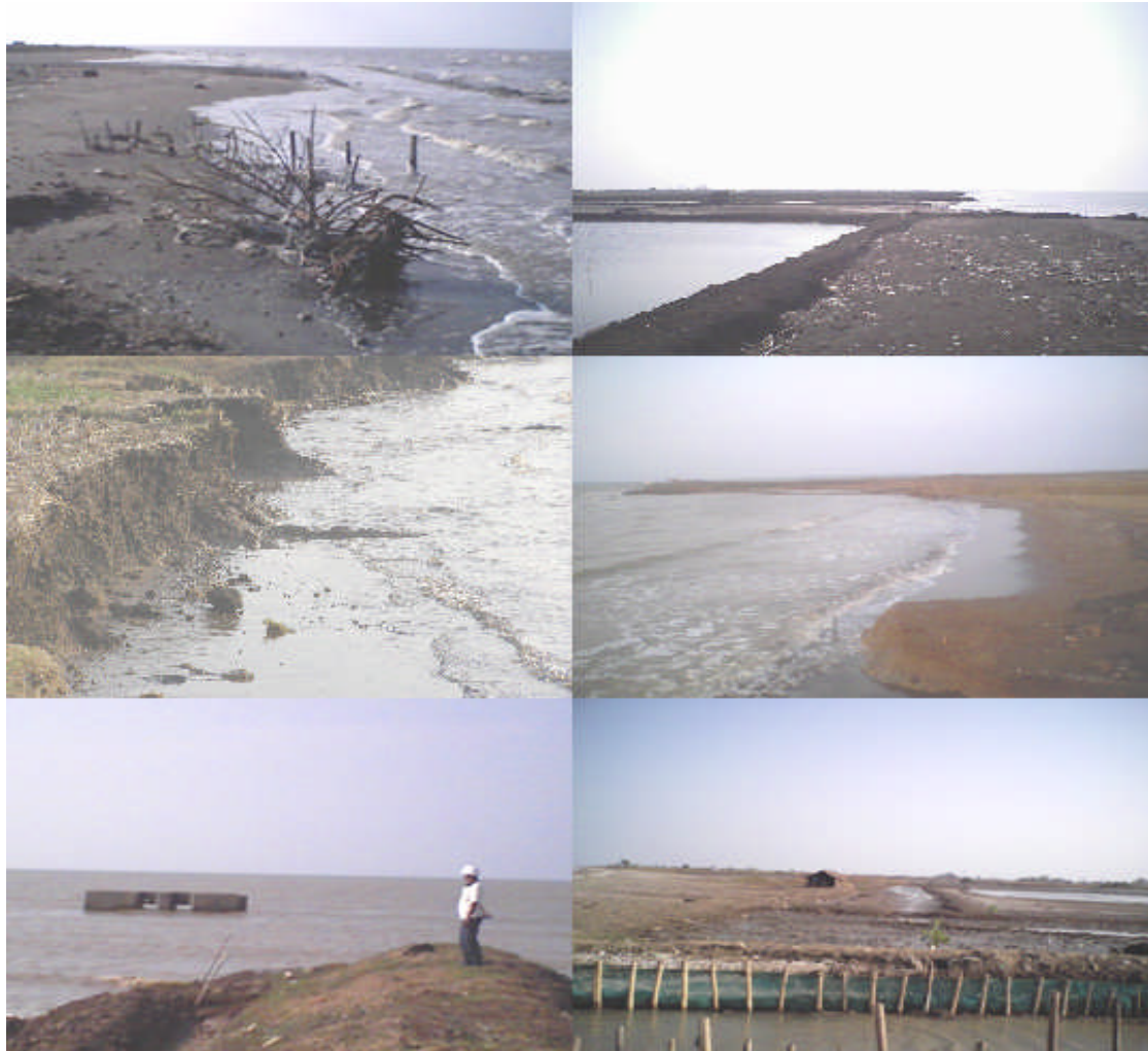
Figure 6. Photos of land erosion in coastal Indramayu
