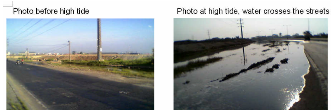
Figure 5. Disposal on Arterial Roads that Causes Overflow onto the Highway
