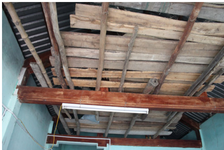
Figure 2: Wooden and bamboo bars are available in most local households in Loc Tri Commune to strengthening their shelter in stormy seasons (Source: Author)
