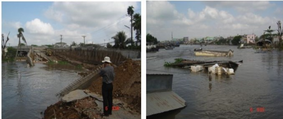
Erosion paths in Tra Nien Bridge Date 03/03/2010 Phong Dien district, length 100 meters, 20 meters deep, eroded 03 apartments, 02 dead
