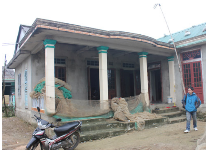
Figure 4: A safe house built by DWF in Thua Thien Hue (Source: Author)
