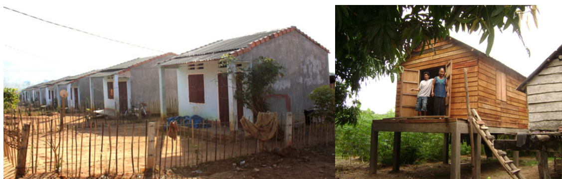
Figure 3: Post-typhoon houses built by VNRC in Gia Lai (right) and Kon Tum (left)
