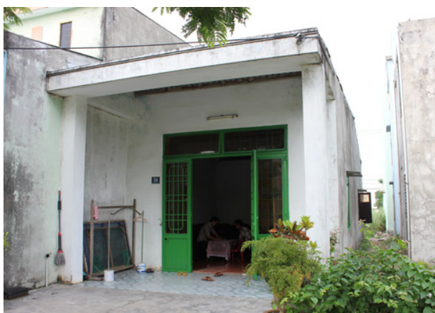
Figure 6: A cyclone-resistant house built in support of ISET in Da Nang (Source: Author)
