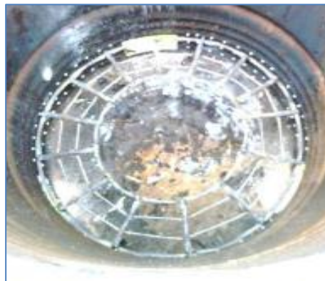
Figure 5: Fire grate at the bottom
