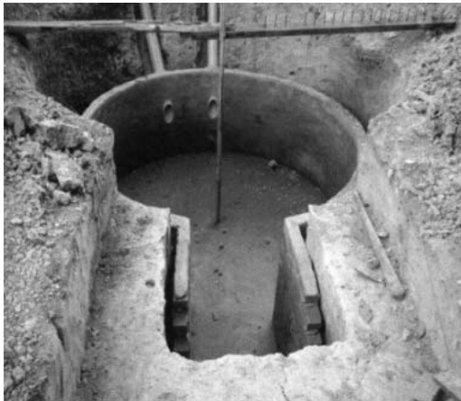
Figure 4.11 Digester (Photo by LBPP)
