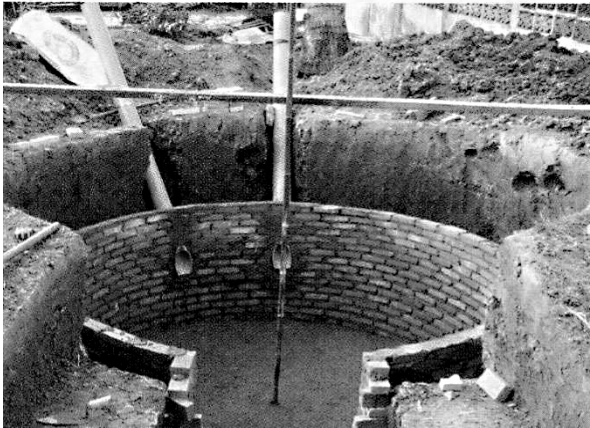
Figure 4.10 Inlet pipe (Photo by LBPP)
