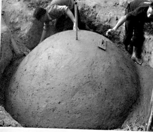
Figure 4.12 Gas storage tank (Photo by LBPP)
