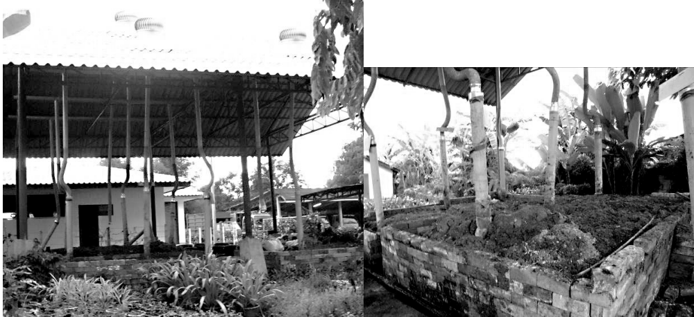
Figure 4.4 A static aerated composting system in Muangklang Municipality Thailand
