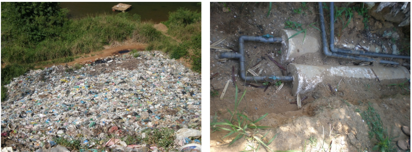
Figure 9. Open landfill next to the the Mahaweli River (left) and in-situ landfill leachate treatment which is undertaken by the University of Peradeniya (A research project lead by Dr Mowjood) (right).
