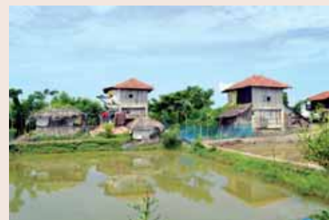
Image 2: Disaster resilient houses in Shyamnagar (Source: Kabir, 2017)
