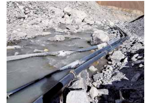
Figure 2: Pipelines to siphon water
