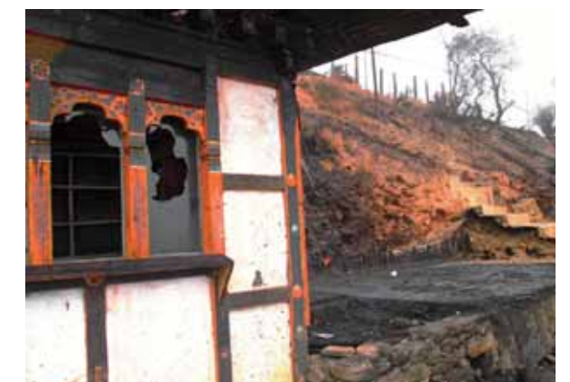
Figure 2: Premise destroyed by fire
