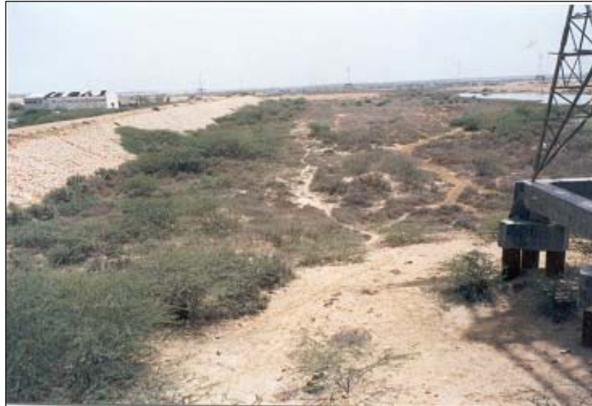
Figure 8: Flood protection embankment on the left side of the Malir river
