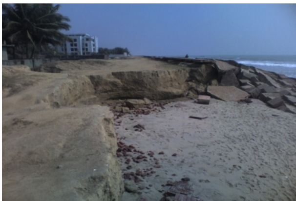
Figure 3. Erosion and land sliding in Cox's Bazar, Bangladesh
