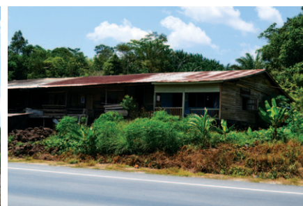
Figure 3. Long House—a long house near Dalat, Selangau, in Sibul District. Area nearby is a vast stretch of privately-owned oil palm plantations
