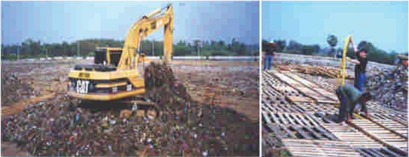
pallet built ventilation system
