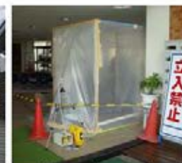
Measuring at the workspace gate
