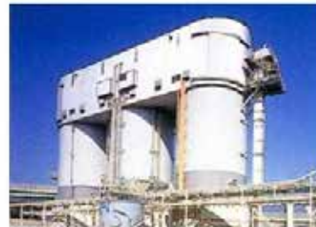
Gypsum storage silos
