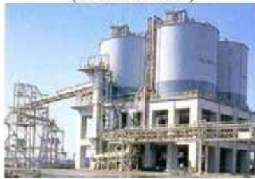
Coal ash storage silos
