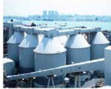
Coal silos, enclosed belt conveyors
