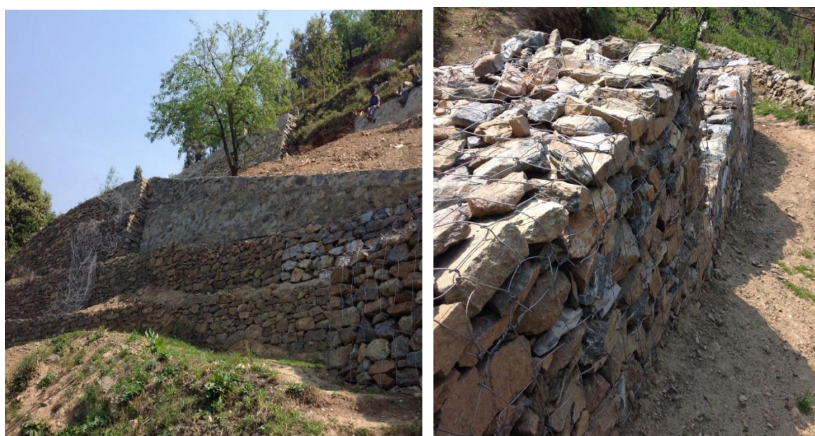
Retaining walls and drainage culverts Ramgad watershed (photo: Lance Heath)
