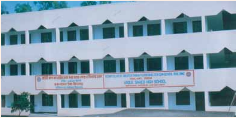
Rotary Club of Greater Dhaka Flood Shelter-cum-School Building, Savianagar, Kisorgani, Bangladesh
