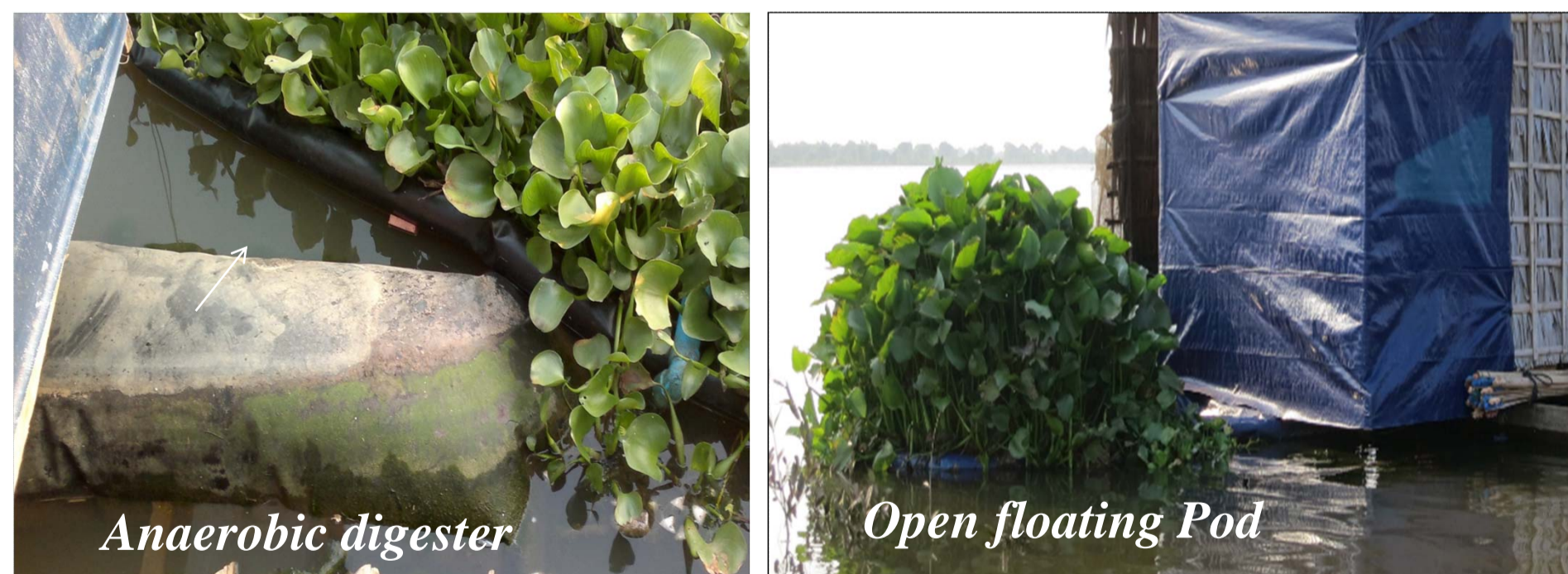
Figure 2. The HandyPod contains and treats household wastewater to a level safe for recreational use.
