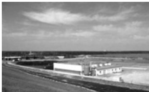
Figure IV.3 A BEKON dry digestion plant
