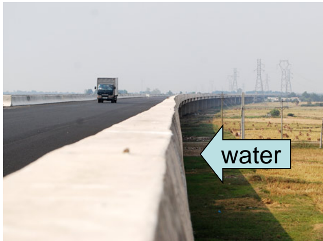
Sky way allowed water moving on the ground
