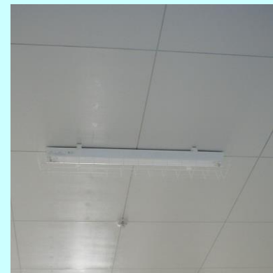
Calcium silicate boards containing asbestos Asbestos cement slates (ceilings)
