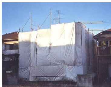
Example of work curing tube-and-coupler single-row scaffolding with flameproof sheets
