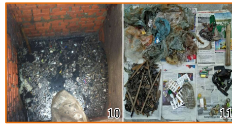
Waste deposition in the manhole (10) and waste components deposited in the manhole after washing (11).
