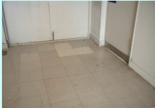
Vinyl floor tiles containing asbestos (floors)
