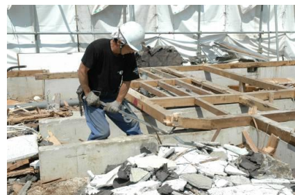
Removing sills
