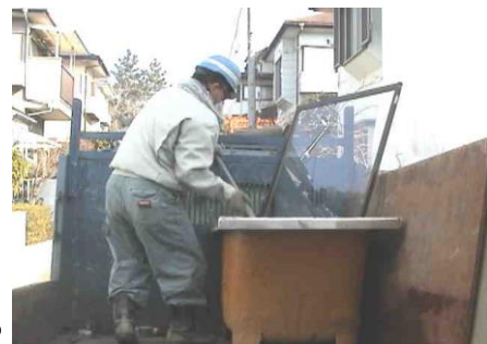
Breaking window glass using a bathtub
