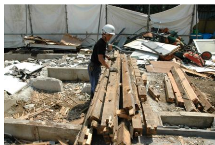
Accumulating CCA-treated wood
