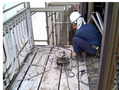
Removing a balcony made of metal
