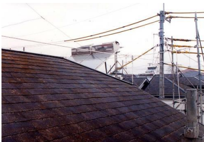
Rooftop-installed object (solar water heater)
