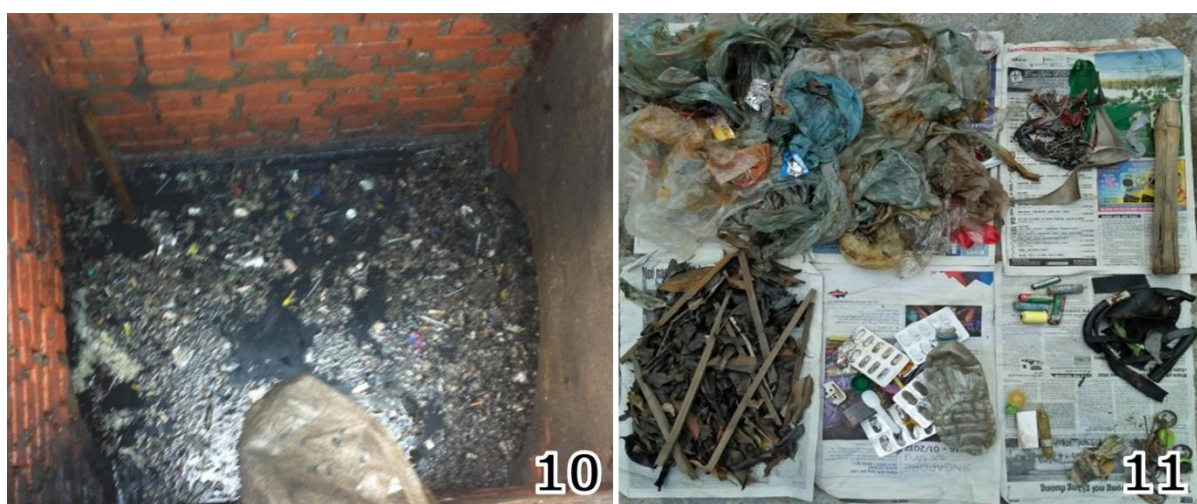
Figure 18. Waste deposition in the manhole (10) and waste components deposited in the manhole after washing (11).
