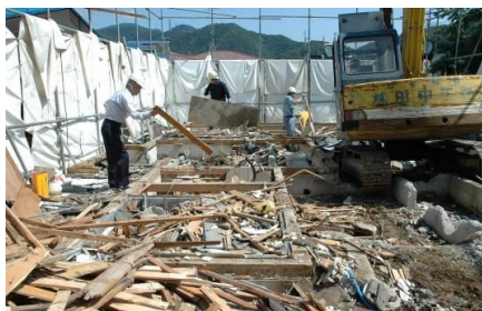
Situation after demolishing upper structural parts with foundations being left
