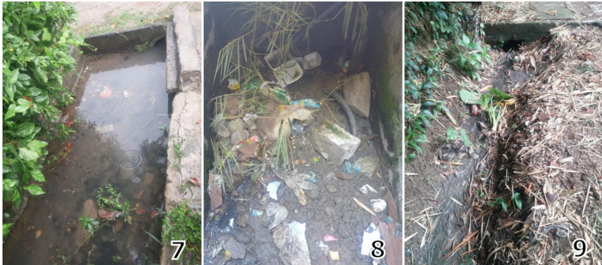
Figure 15. The waste in the open drainage systems at Mang Ca Nho (7), Nguyen Chi Thanh (8) and Nguyen Binh Khiem streets (9).
