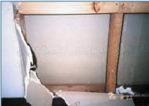
Gypsum boards containing arsenic or cadmium
