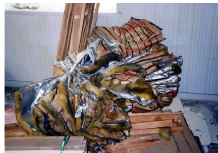
Heat insulating materials being bundled
