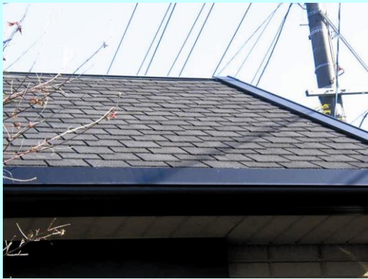
Decorative slates for house containing asbestos (roofs)
