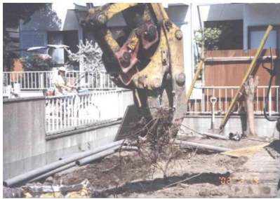
Removing a septic tank
