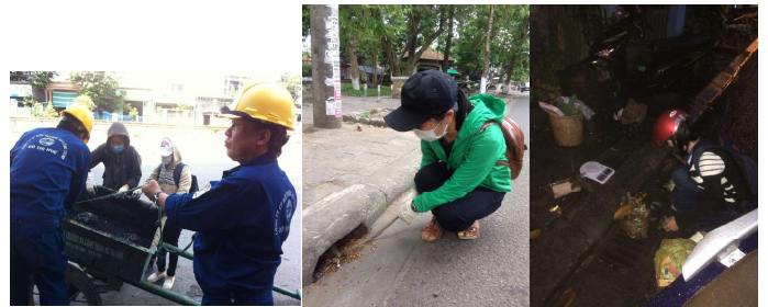
Waste sampling in throats, open drainage systems and the manholes
