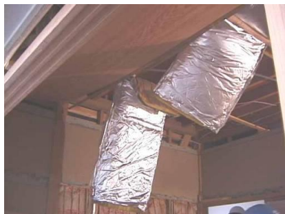
Heat insulating materials being removed
