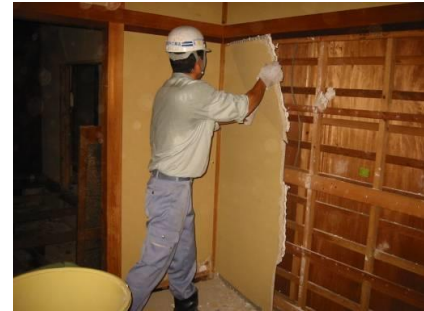
Removing gypsum boards
