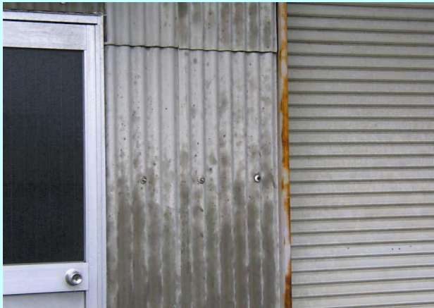
Asbestos cement slates (roofs and exterior walls)
