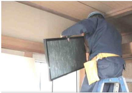
Removing inner fittings
