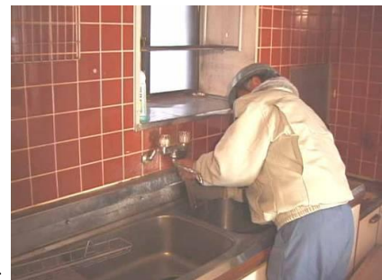
Removing kitchen cabinet and sink
