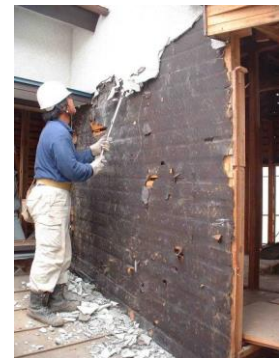
Demolishing a mortar exterior wall
