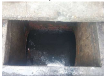
Waste in manholes
