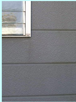
Asbestos boards (ceramic siding)
