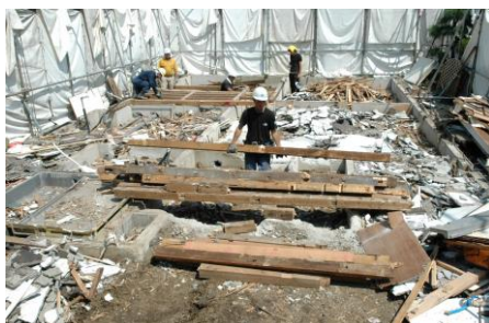
Carrying CCA-treated wood by hand work
