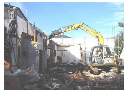
Demolition work of outer peripheral parts by the overturning demolition method
