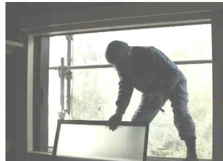
Removing external fittings (window glass)
