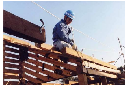
Removing joint metals
