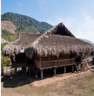
Traditional Bamboo Roof
