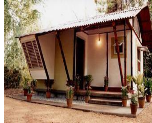
Figure 5: Demonstration House by IPIRTI- Bangalore, March, 2001
