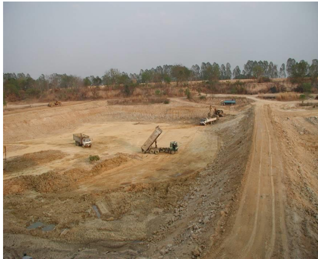
Figure 2.10 Sanitary landfill under construction
