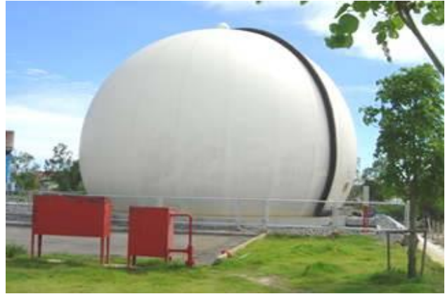
(b) Gas collection tank
