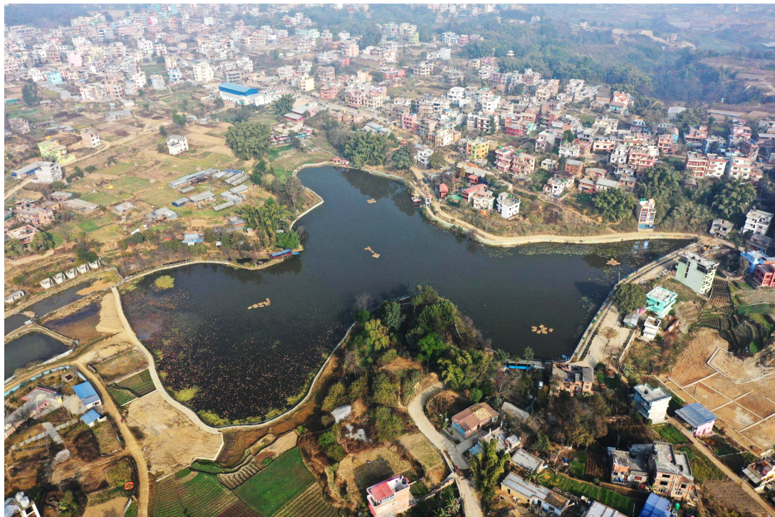
FIGURE 2. Aerial view of the Nagdaha with the installed floating rafts and the settlements around it (Photo credit: Samyak Prajapati, SEN).
