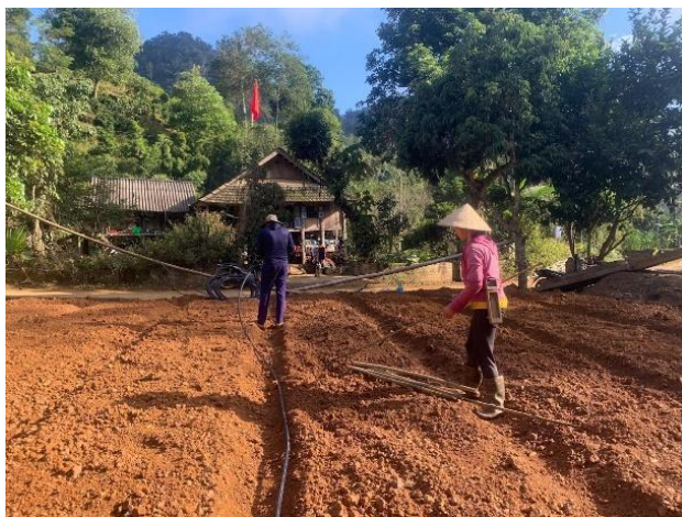
FIGURE 7. Installing irrigation systems for households.
