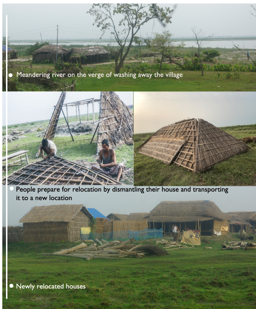
FIGURE 4. Adaptation to a meandering river. Local communities begin relocating when the river threatens to wash away their houses. Houses are constructed primarily from locally available materials and designed to be easily disassembled, transported by a few people, and reassembled at a nearby, safer location.
