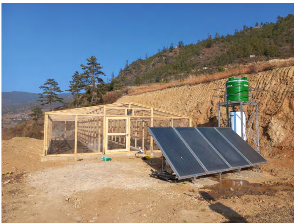
FIGURE 1. Smart greenhouse developed in the temperate region with SWHS as the heat source.
