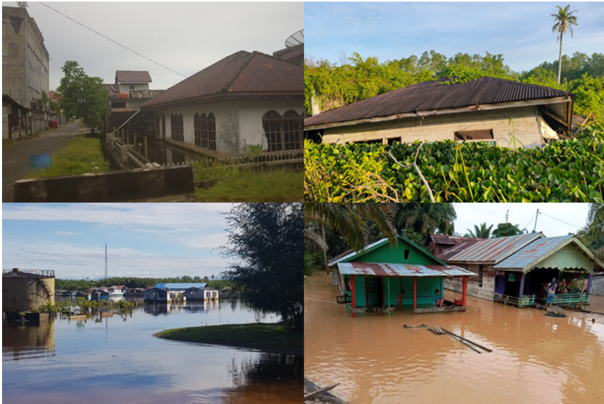
FIGURE 3. Singkil coastal area is experiencing worsening flooding due to land subsidence (bottom). Houses have been damaged and abandoned due to the land subsidence and liquefaction (top).
