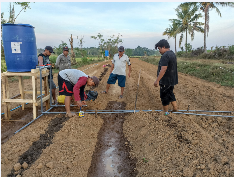
FIGURE 11. Connecting lateral pipes.
