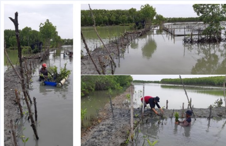
FIGURE 12. Demonstration site development.
