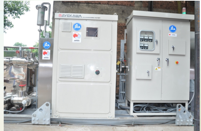
Demonstration unit of Electric Heat Pump (EHP) in a milk dairy
