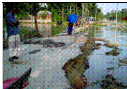
Figure 6: Flood Damage Pavement
