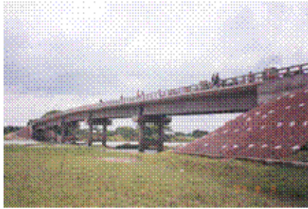
Figure 7: Span increased and approach strengthen
