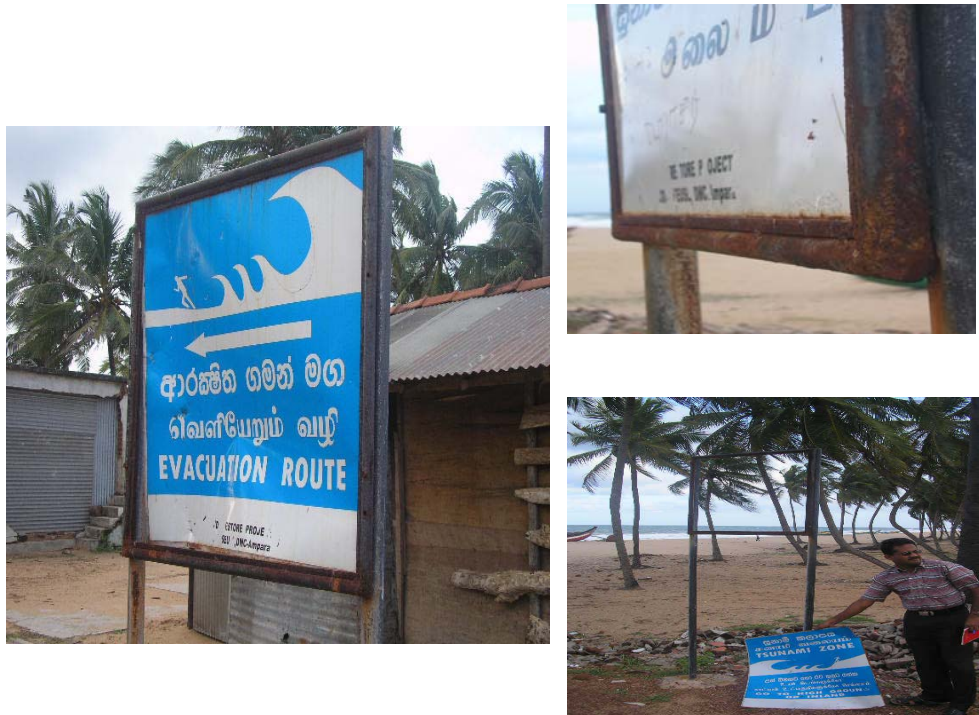
Figure 4: Corrosion and damaging the sign boards
