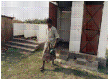
Figure 9: Raised toilets and water supply system
