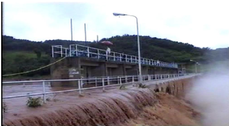
Fig.22 Overflow from the Namtha Dam (7 August 2006)
