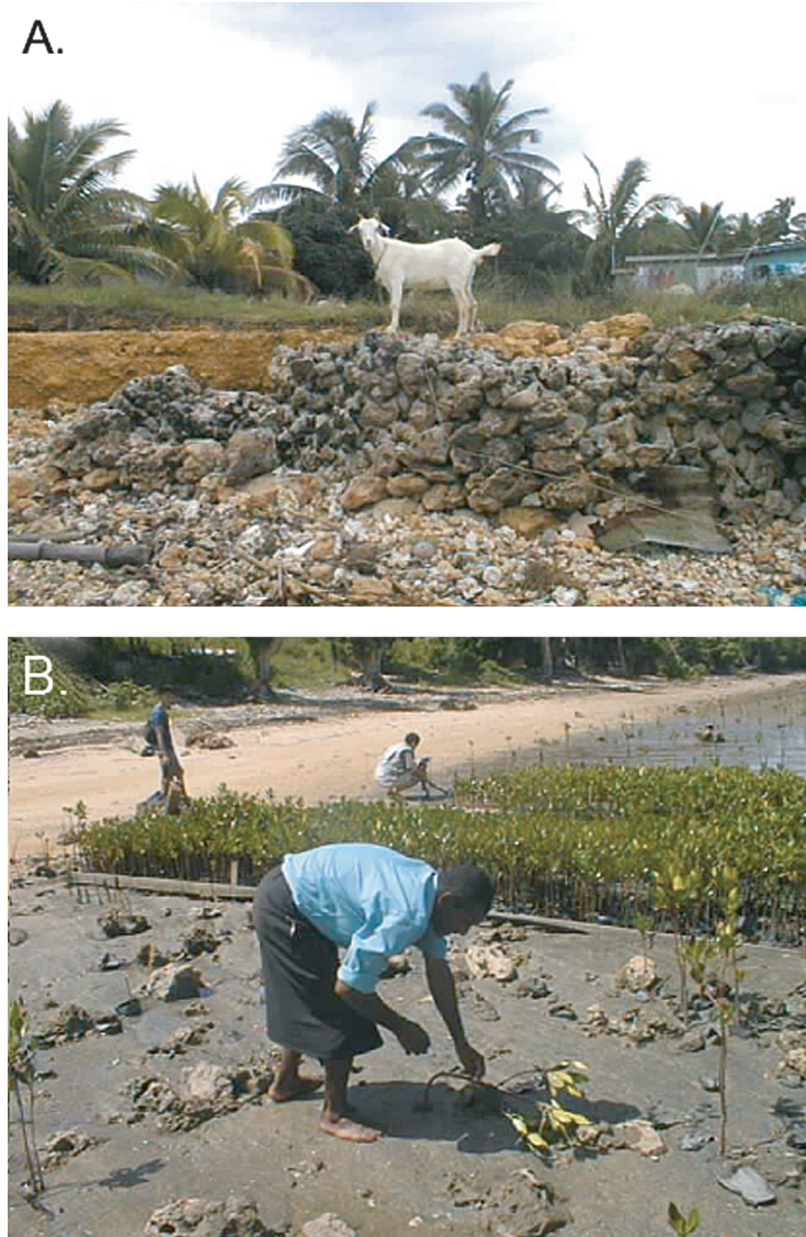
Figure 6.8. Adaptation to erosion along an island shoreline at Yadua Village, Viti Levu Island, Fiji [photos: Patrick Nunn]. (A) The earliest response was to build a seawall using largely rock from the fringing coral reef. The seawall was undermined by wave erosion, collapsed, and rebuilt repeatedly until it became clear that this approach was not an effective long-term solution. This view shows part of the degraded seawall and the land behind it. Storm waves often impact this coast and erode the coastal flat on which the village lies. (B) The villagers are now replanting a mangrove forest along the worst affected part of the shoreline. This option is sustainable, effective and enhances the nearshore ecology. The main challenge with this strategy is that it may take 25 years for the mangrove fringe to reach maturity. Mangroves are grown in a nursery (pictured in middle ground) and then planted at regular intervals when they are about 80 cm tall
