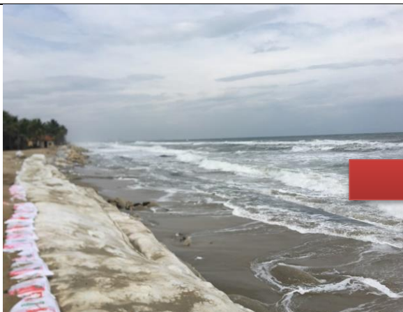
Soft embankment with sand bags - geobags, big sand bags (approximately 80,000m 3 ) in Cua Dai sea, preventing coastal erosion on Cua Dai sea, 2017
