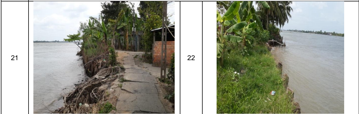
Embankment and rural road in Vinh long city
