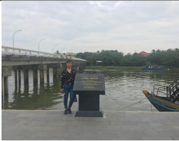
The embankment protects Hoi An ancient town from Cam Nam Bridge to Pagoda Bridge
