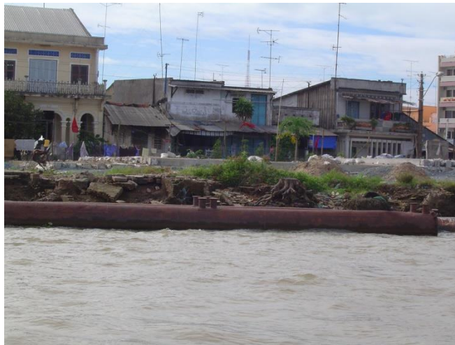
Landslide along embankment of Co Chien River, No.5 Ward, Vinh Long city
