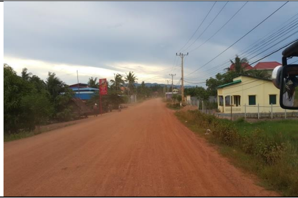
Road/rural road in Treuy Koh Commune (Kampot district). This commune is located close to the coastline. Most commune roads are of concrete or laterite constructions, and are vulnerable to flooding during the rainy seasons
