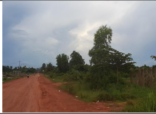
Road/rural road in Treuy Koh Commune (Kampot district). This commune is located close to the coastline. Most commune roads are of concrete or laterite constructions, and are vulnerable to flooding during the rainy seasons
