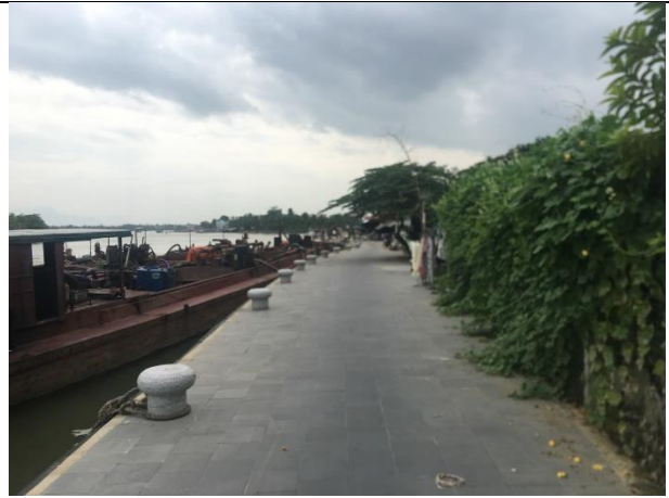
5m wide Larsen concrete sheet pile embankment. Embankment aimed at protecting Hoi An ancient town from Cam Nam Bridge to Pagoda Bridge
