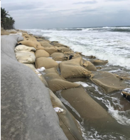
Soft embankment with sand bags on Cua Dai sea, preventing coastal erosion on Cua Dai sea
