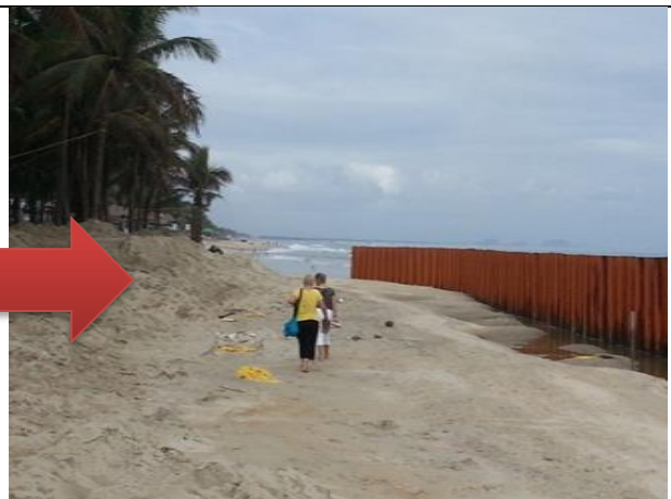
Temporary embankment with metal sheet, breakwater, 2014
