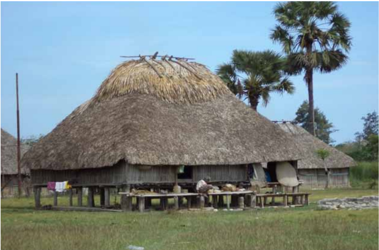
Figure 2.3.2: Traditional house in Raimea Village, Covalima, Timor-Leste, with Ai Tatan to clamp the roof from storms and strong winds, and Lenik to prevent strong winds from entering the house.
